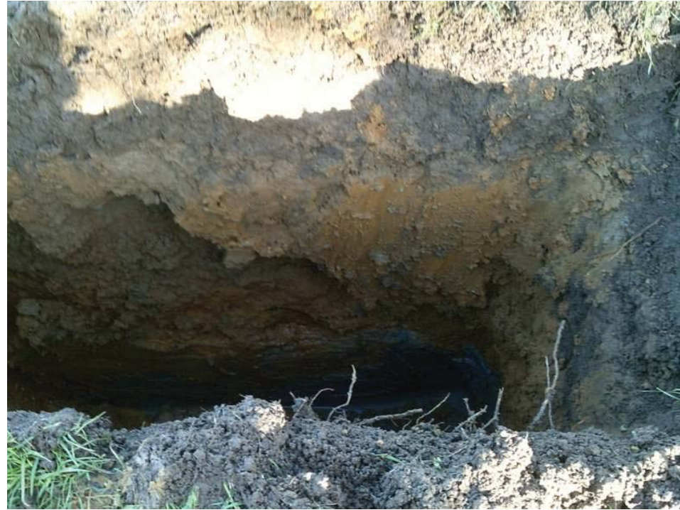
Trial pit 09 west face
