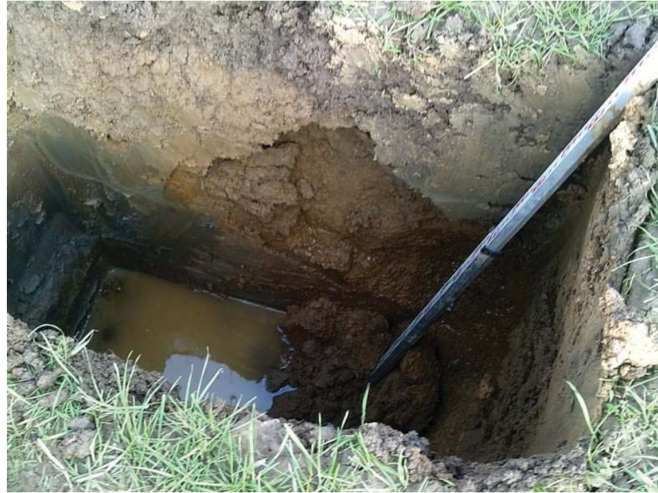
Trial pit 07 north face
