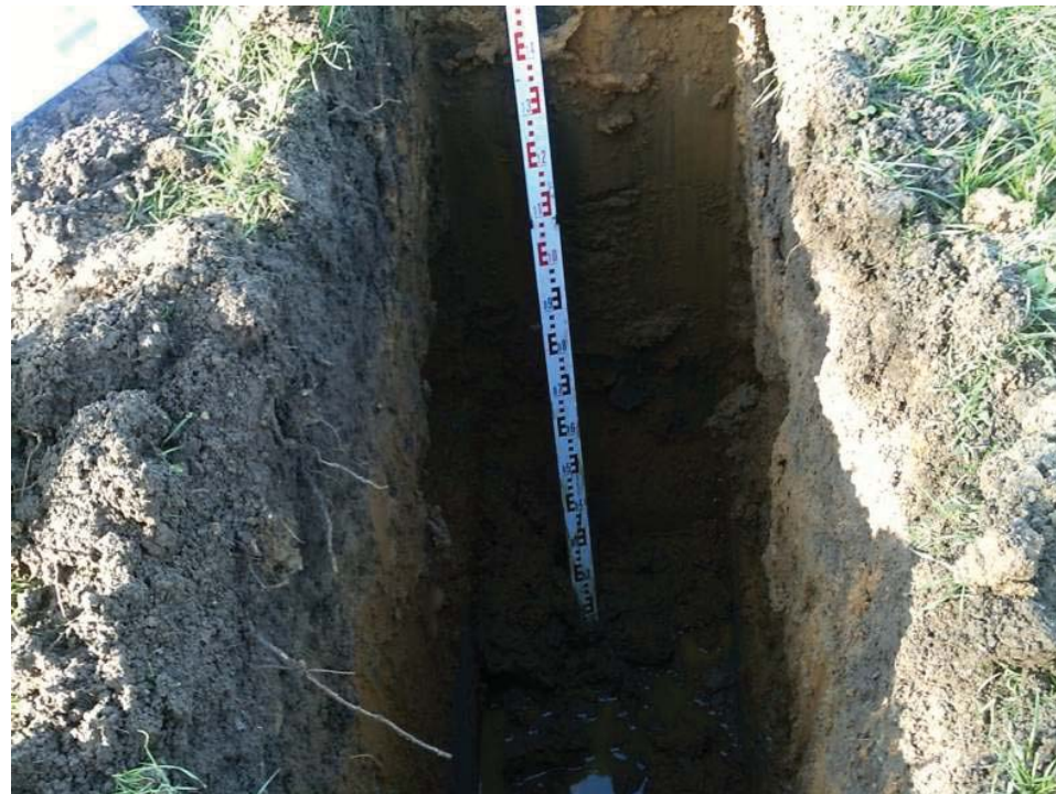
Trial pit 09 south face
