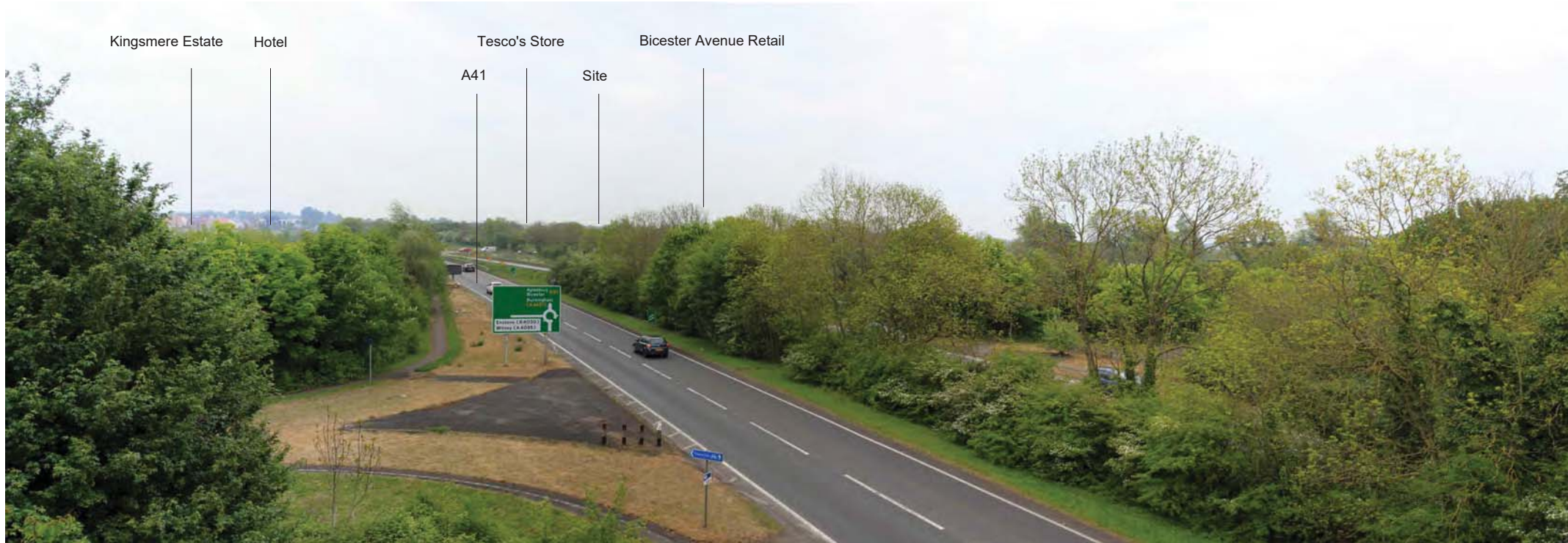
View Location 5 - From A41 overbridge looking north east
