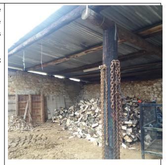
B5 to 8 were of similar construction and comprised of open barns, constructed of wooden beams and metal corrugated sheets.
