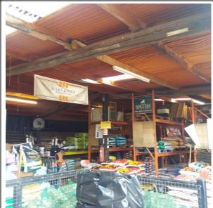
B3 comprised of a storage building constructed of limestone bricks, wooden beams and a metal corrugated roof. It appeared to be former stables. No obvious roosting points were located and it appeared well sealed.
