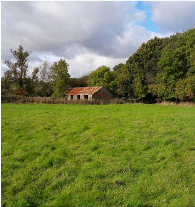
Figure 12 – View of Home Farm Barn from the access track.
