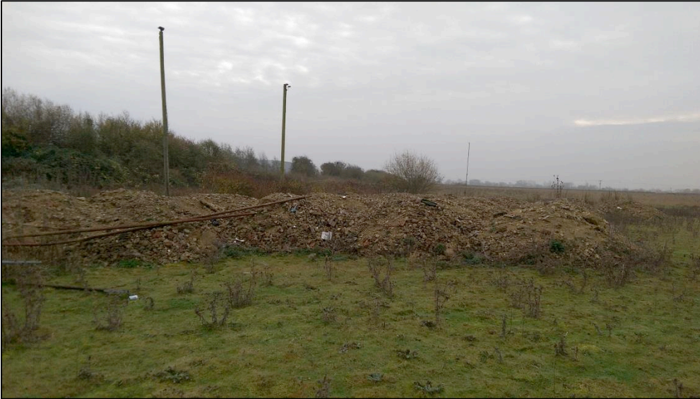
Plate 3: crushed concrete piles in North East Corner
