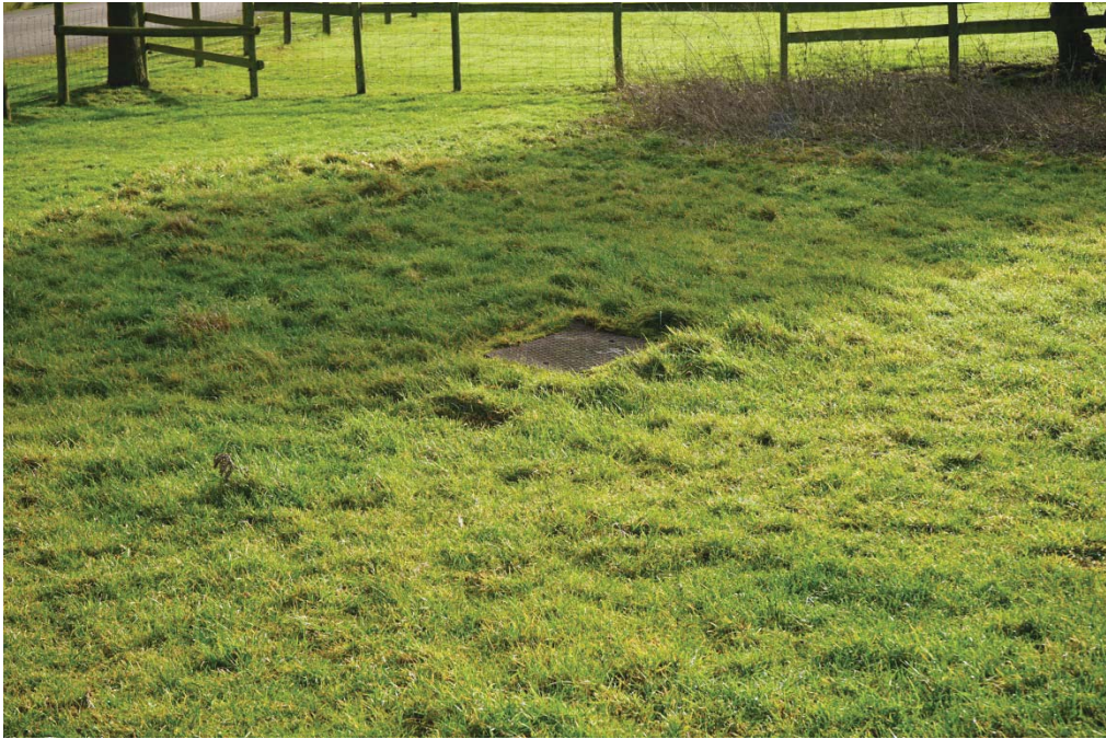
Plate 8: Manhole seen within the site, for drainage to the filter bed.
