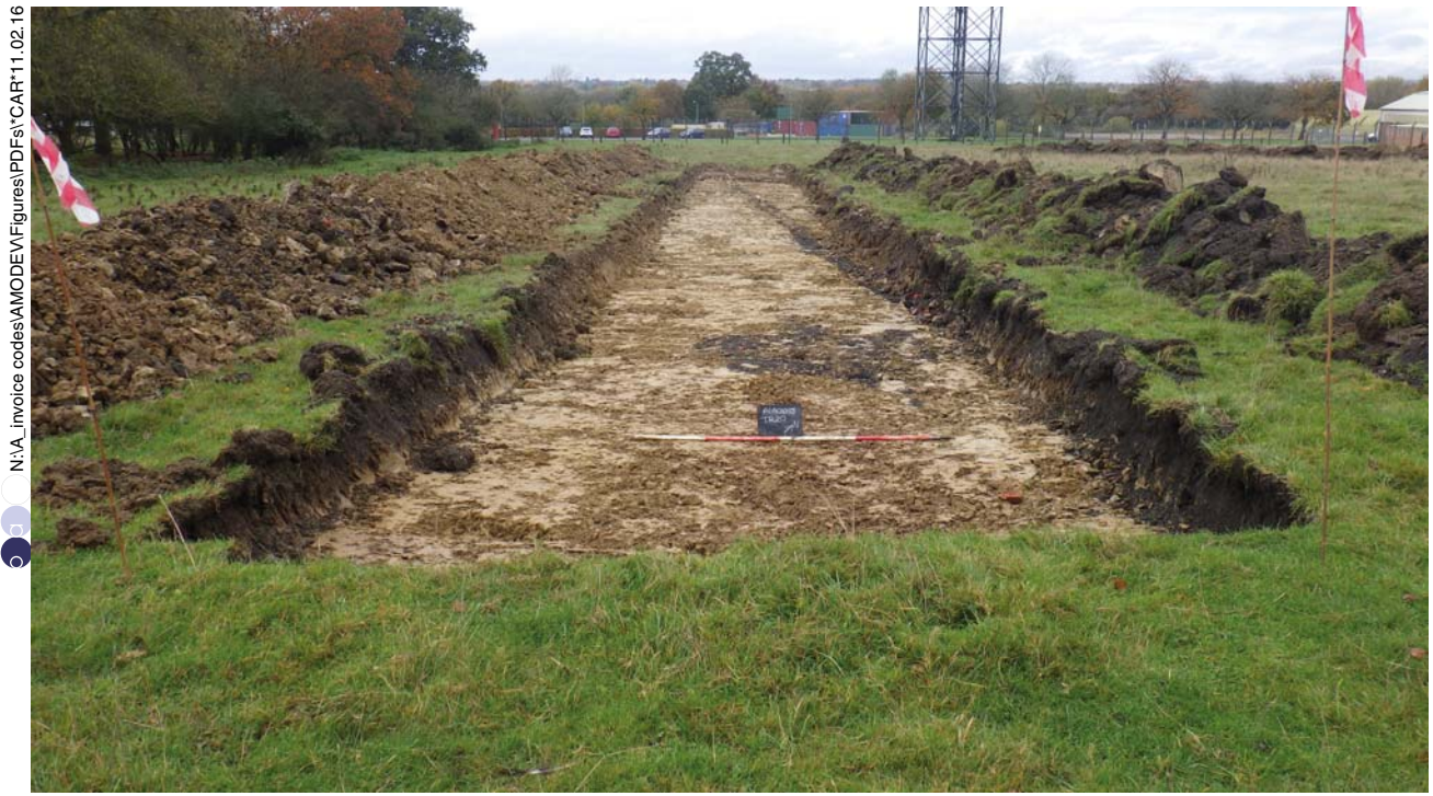
Plate 8: Trench 20 View of military camp related demolition debris
