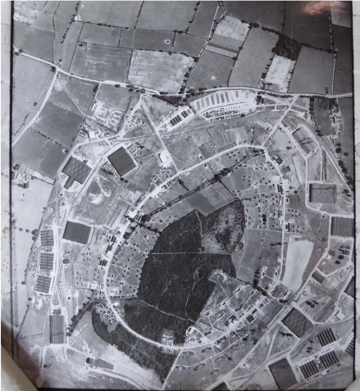
Plate 7: Aerial image of the military camp in 1945 showing the newly constructed large warehouse buildings and camp hut accomodation units
