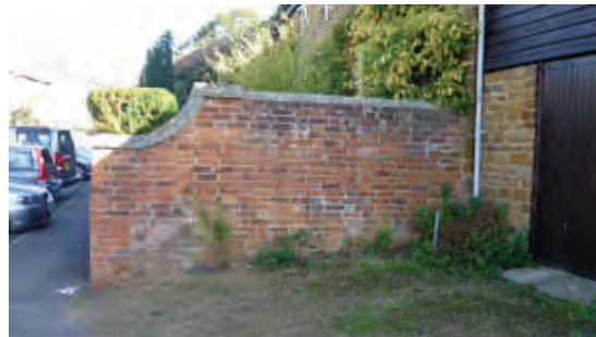
Side boundary brick wall with sweeping coping adding interest to the streetscene
