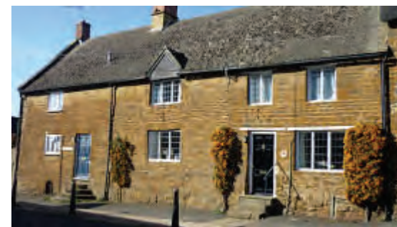
Corner Cottage and Beggars Roost: both have stepped entrances indicating the steep slope towards the church
