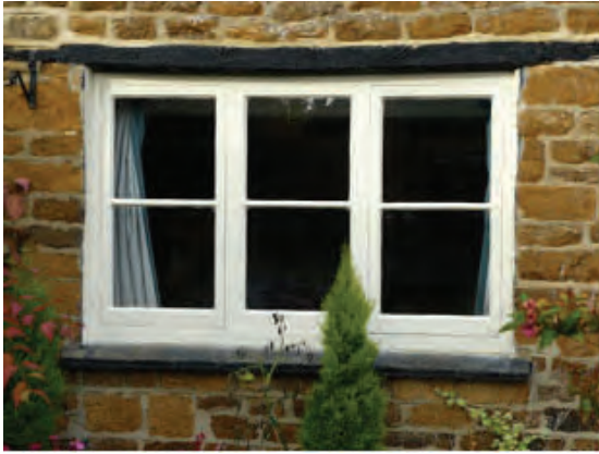
Good example of a replacement of a traditional flush timber casement
