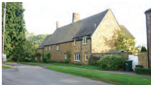
1 and 2 Manor Road: no.2 (right) has been altered more than no. 1, creating windows on the north elevation which are larger than the traditional openings next door
