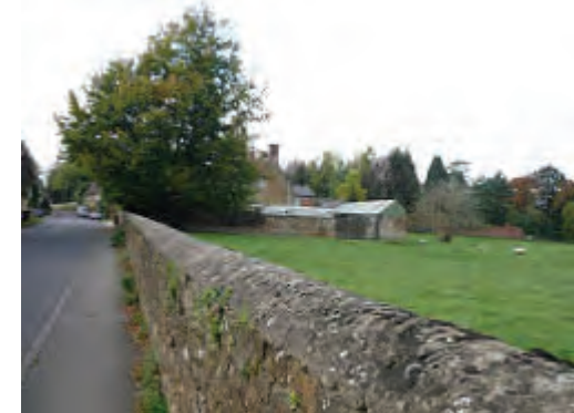
Strong walls mark the edge of Water Lane
