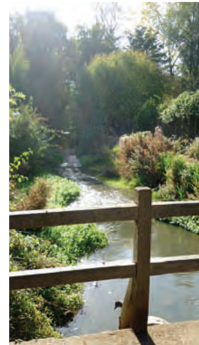
The repaired bridge over the Sor Brook provides a convenient and traditional vantage point to enjoy the stream's progress through the valley
