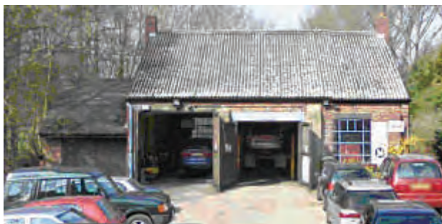
The old pump house
