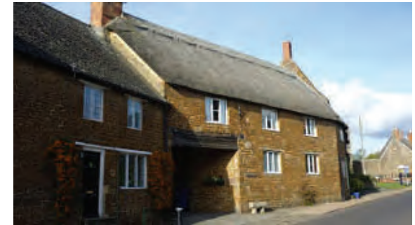
Former Royal Oak public house converted to residential use, preserving the building
