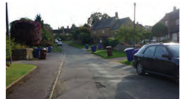
Traditional verges on the right contrast with the modern footway on the left on Tanners Lane
