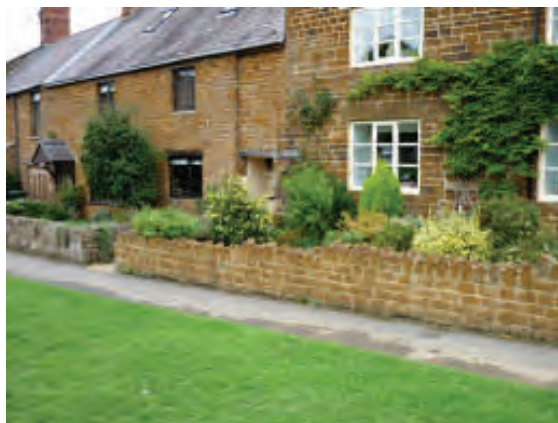
Traditional stone walls outside Tarvers and Verndale maintain boundaries while preserving the streetscene
