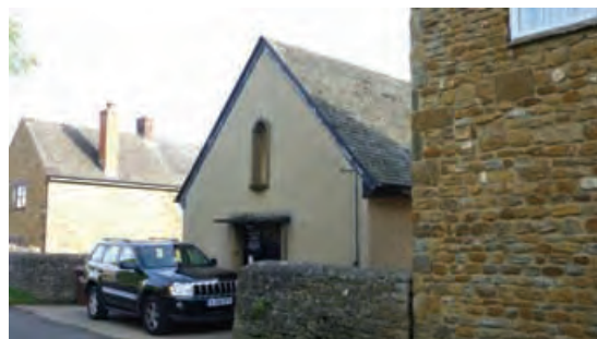
The Roman Catholic chapel on Round Close Road: small but functional and has tried to blend in with the historic surround-
