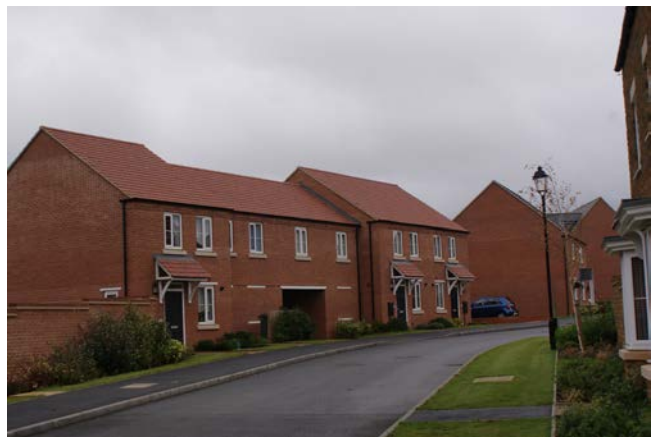
Image 1: Terraced brick units with rear courtyard access
