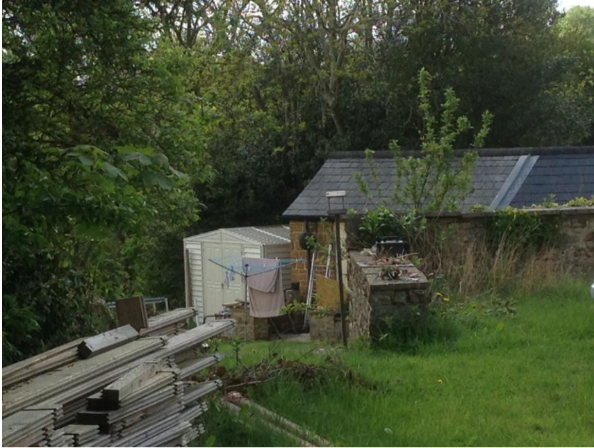
Planking from demolished shed, Summer 2016
