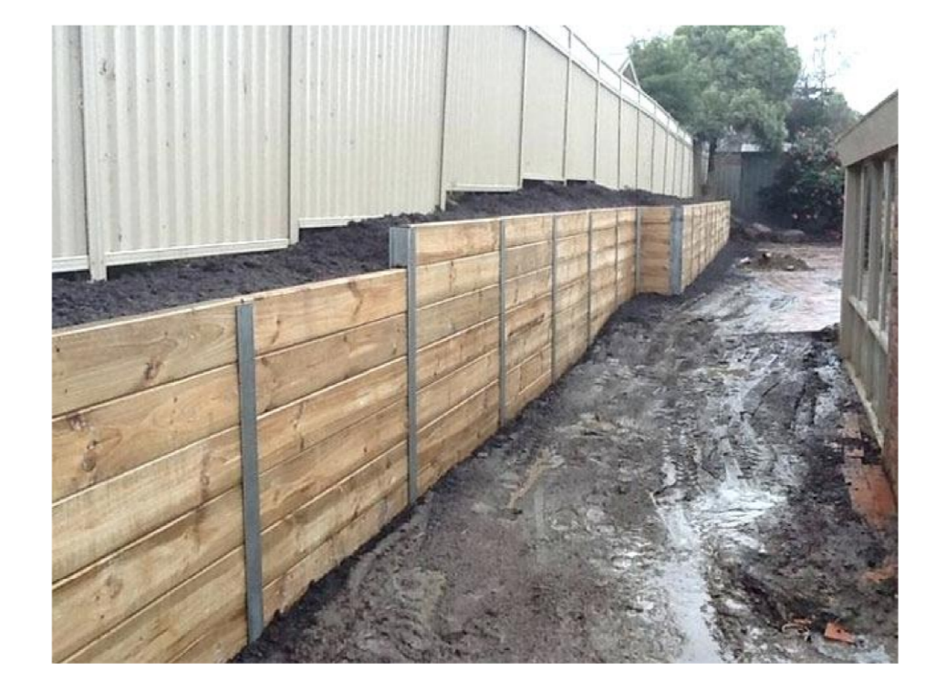
08 TIMBER RETAINING STRUCTURE around substation 1017
