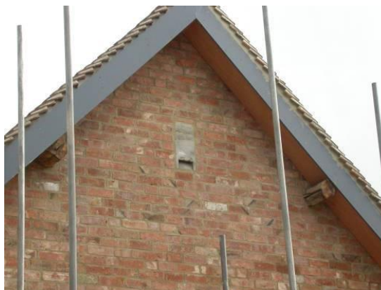
Fig. 7 Bat tube installed in gable end
