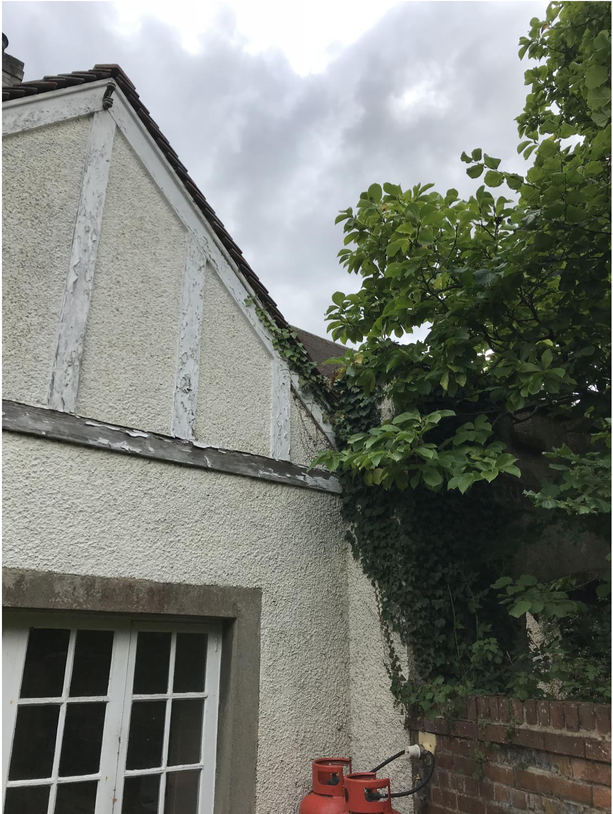
Photo showing new flue location hidden behind existing wall/roof junction
