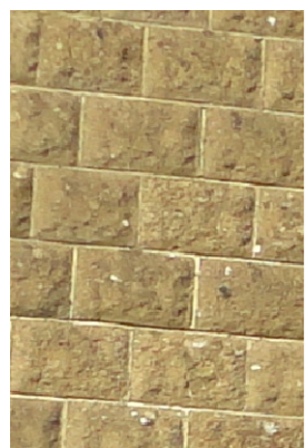
Image of existing concrete blocks
