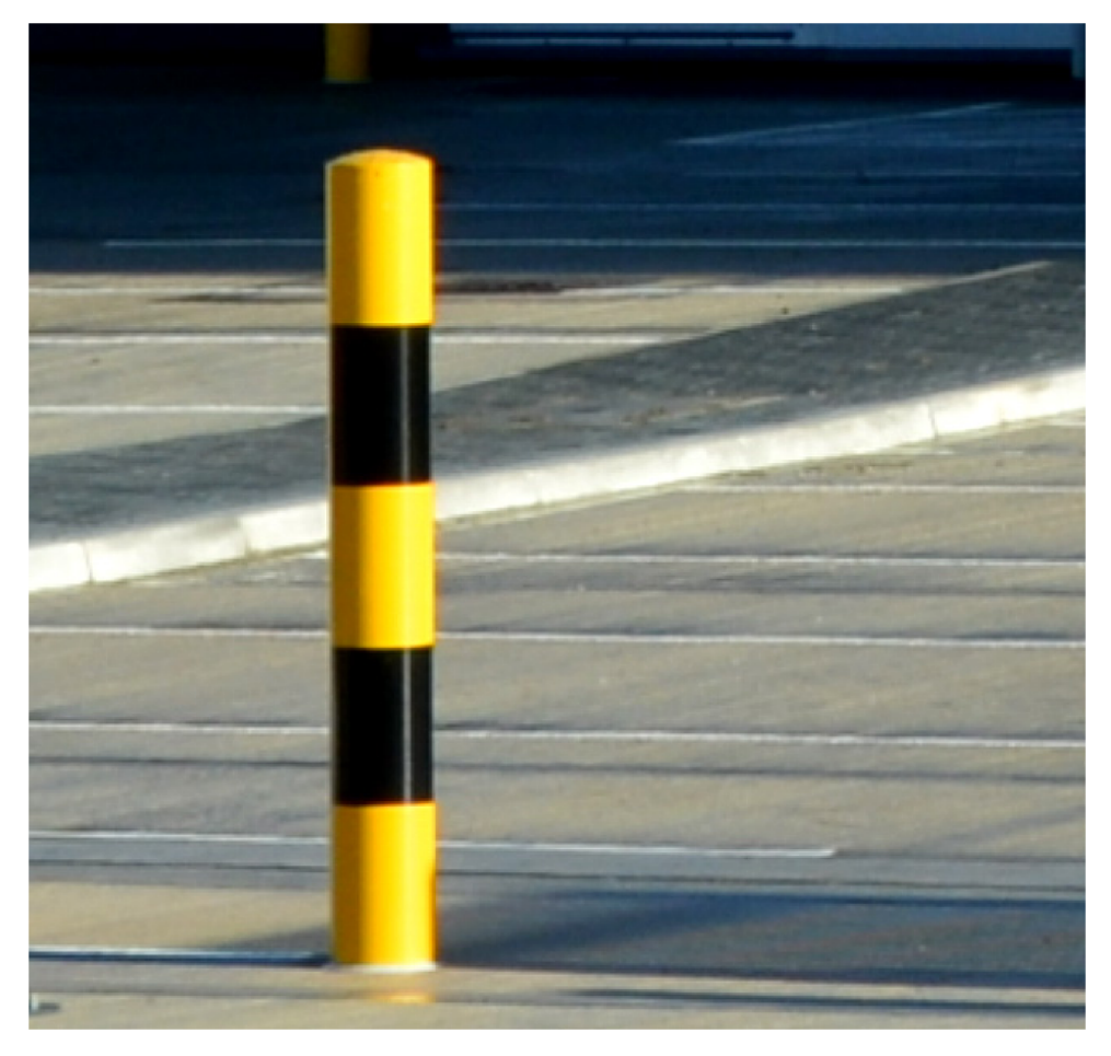
06 PAINTED STEEL PROTECTION BOLLARD 012 at loading doors
