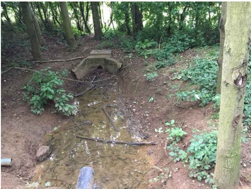
Photograph 4: Inside woodland belt showing existing headwall and ditch
