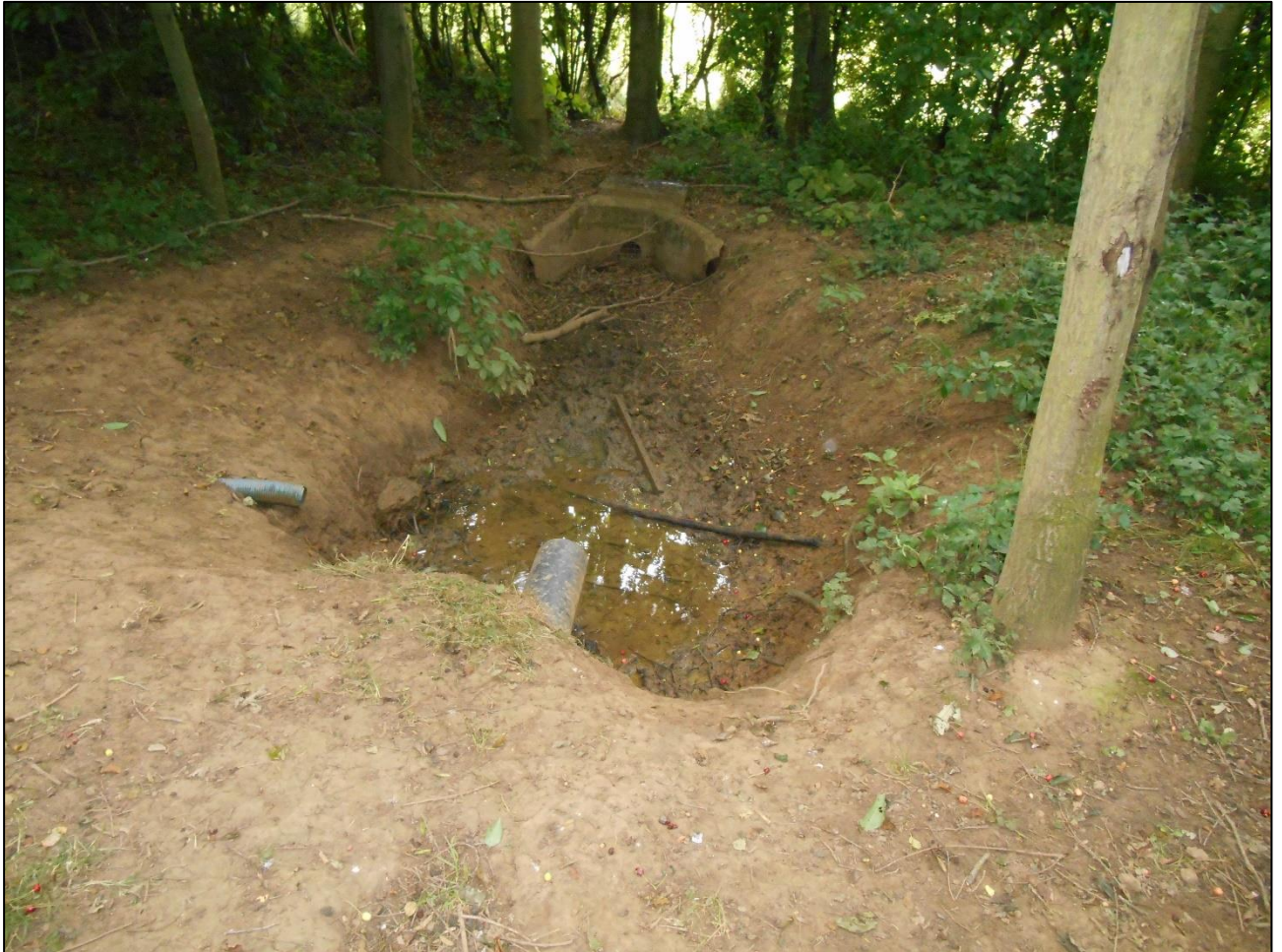
Image 3: part of the existing drainage route across the tree belt
