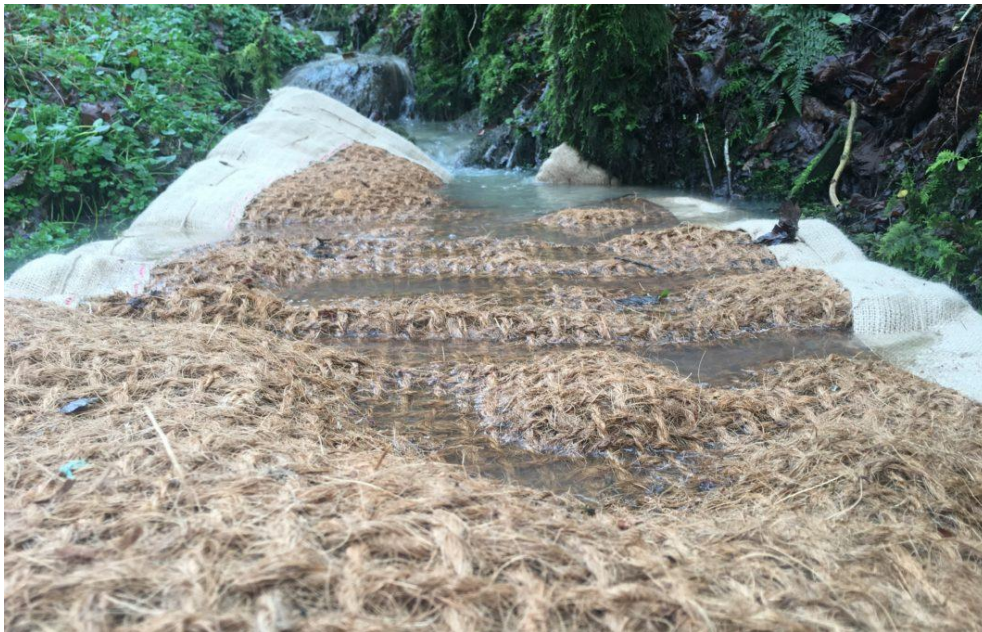
Image 1: Silt mat positioned in watercourse
