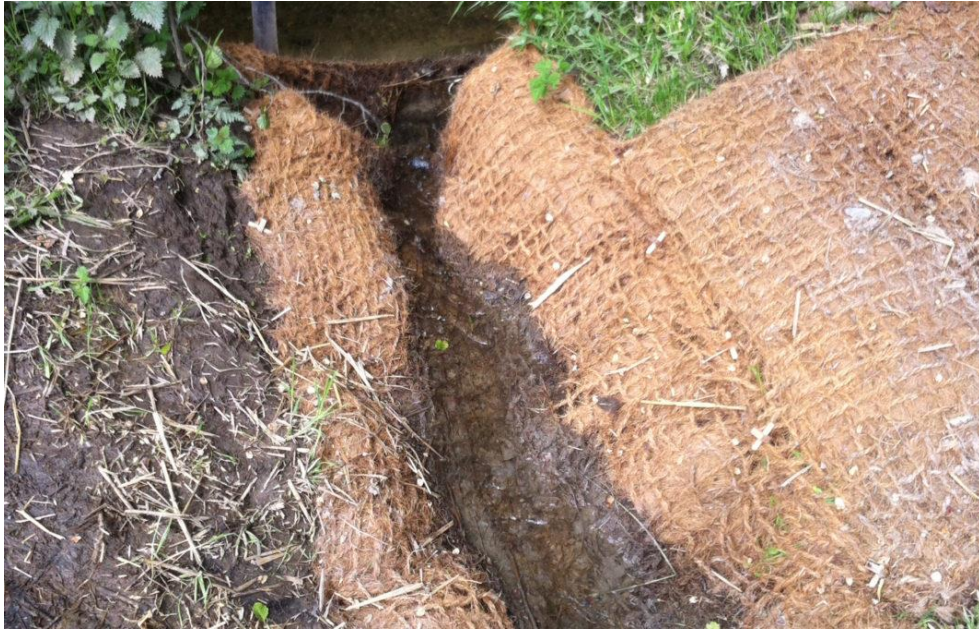
Image 2: Floc mat positioned in ditch
