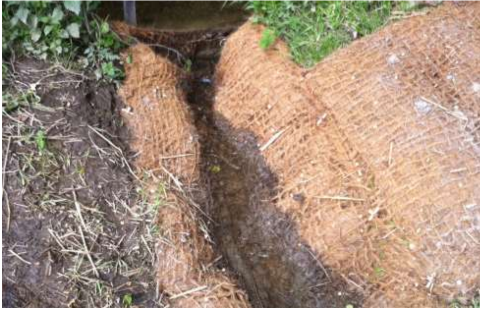
Image 2: Floc mat positioned in ditch
