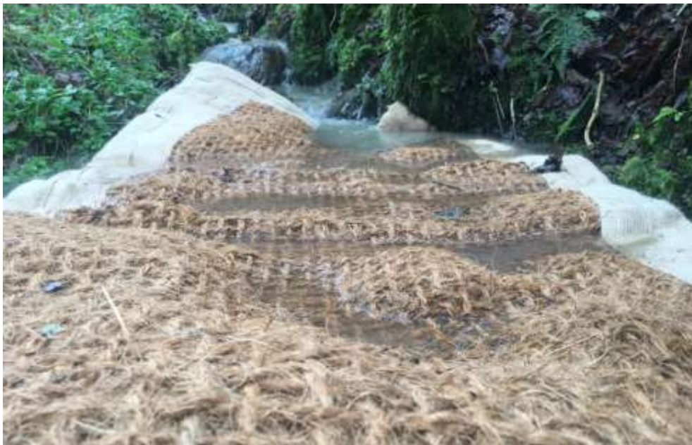
Image 1: Silt mat positioned in watercourse
