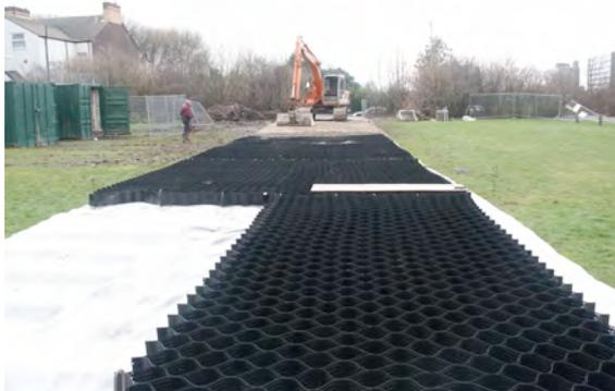
When considering damage to tree roots, in applications of vehicular access and parking, the risk of oxygen depletion caused by compaction of subsoil's, site clearance damaging the root source and type of reinforcement are areas which need to be given due consideration.
