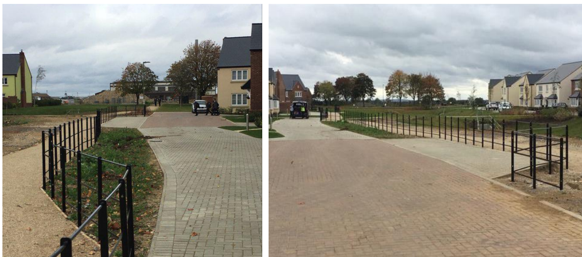
Images showing the railings in situ
