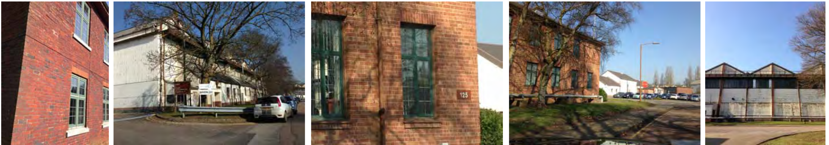
EXISTING TRIDENT AREA BUILDINGS
