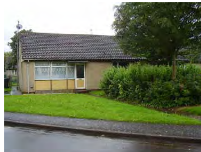
BUILDING 650 TO BE RETAINED
