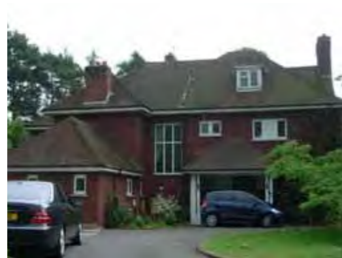
BUILDING 2 TO BE RETAINED
