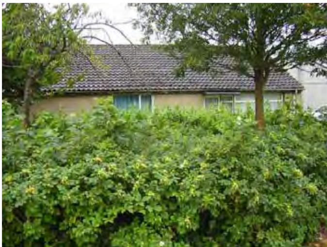
BUILDING 650 TO BE RETAINED
