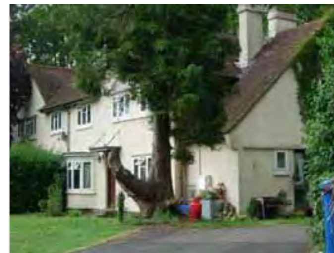
BUILDING 1 TO BE RETAINED
