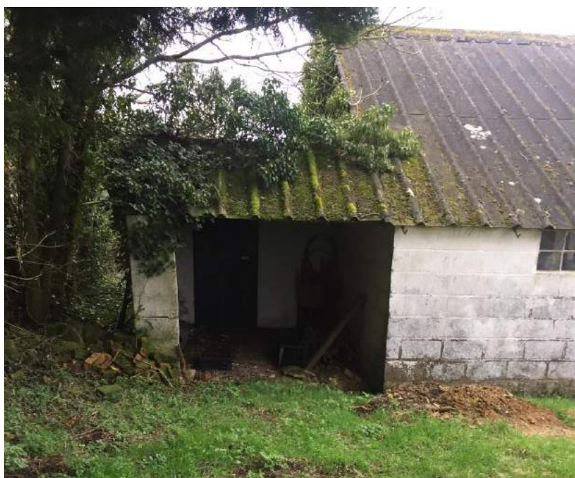
Side entrance to outbuilding (looking south)
