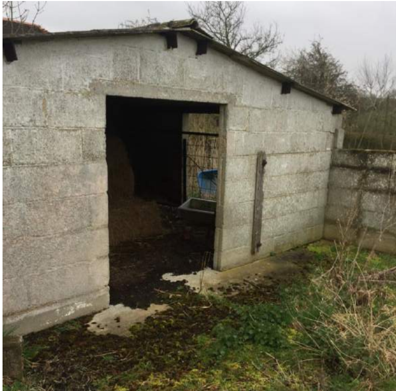
Small outbuilding (looking east)
