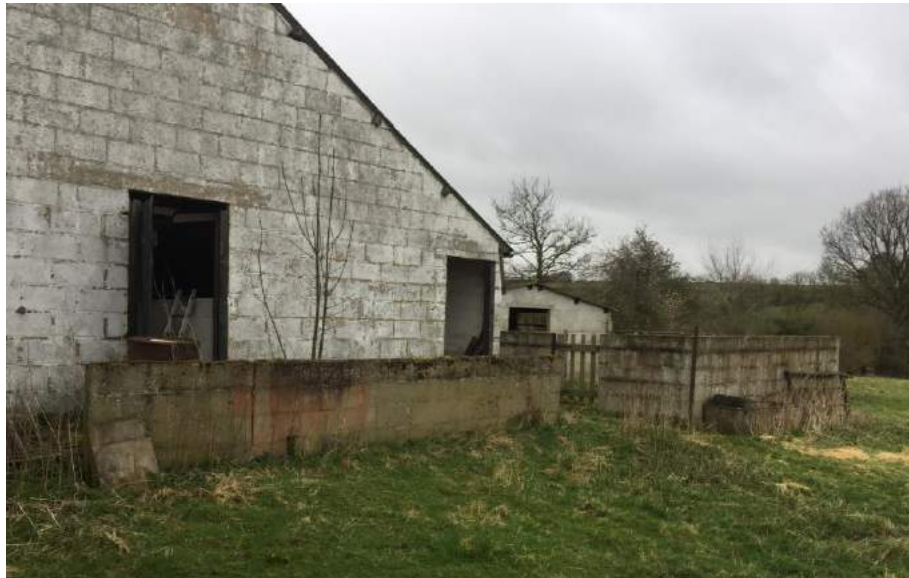
Western side of outbuilding and pens (looking east)
