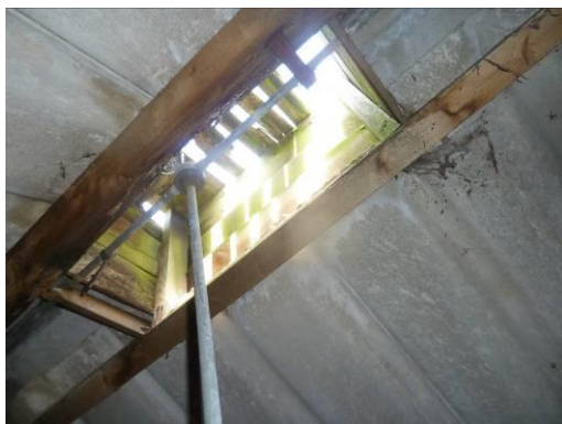
Open air vent in roof
