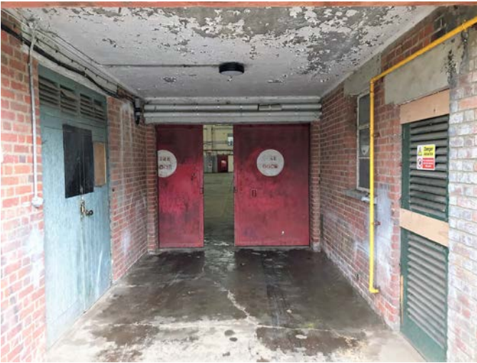
Exterior view of existing sliding steel doors to be retained.
