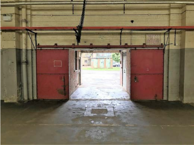
Interior view of existing sliding doors & gear to be retained.
