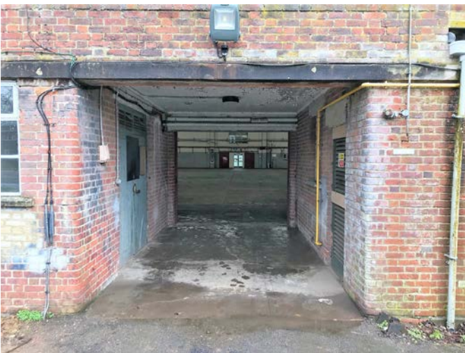
Existing west entrance requiring new fire escape doors.
