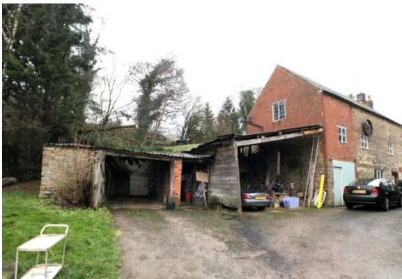
Photo 1: South elevation of the lean to and garage
