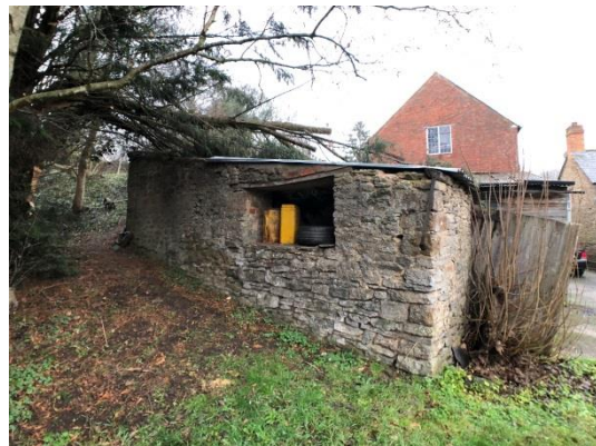
Photo 2: West elevation of the stone garage
