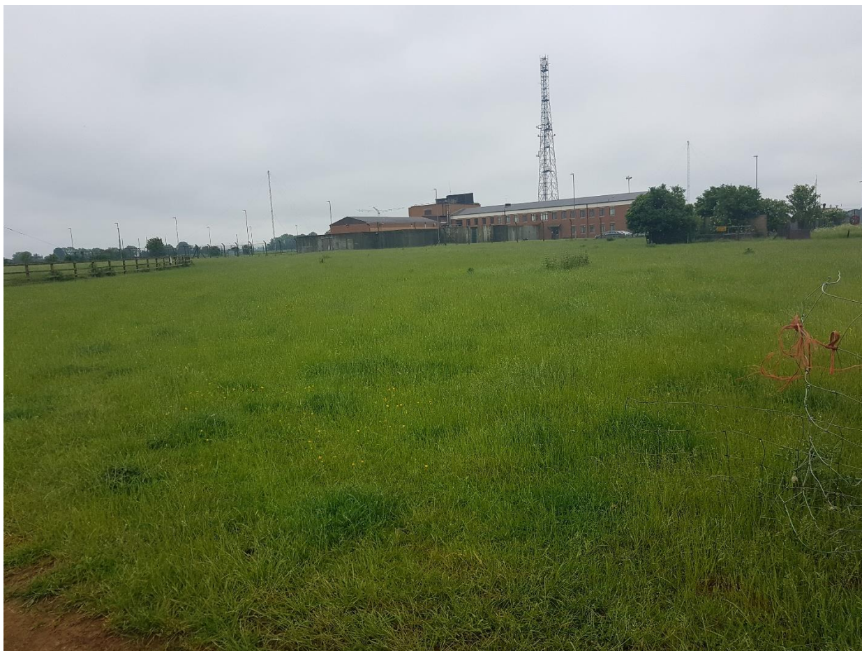
Image 2 – Existing Secure Facility
