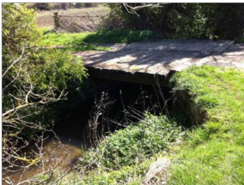
Figure 5 2 – Existing Brookfurlong Bridge
