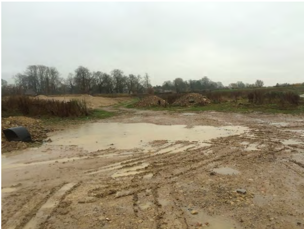
Photograph 1: Earth mounds within Phase 3.
