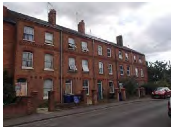
Narrow fronted 3 storey terrace, Banbury
