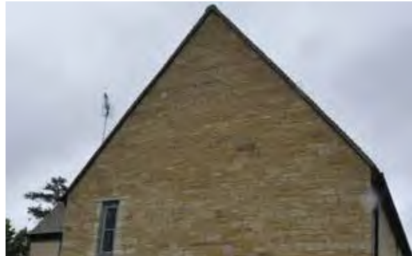
Steeply pitched roof with no overhang, Bletchington
