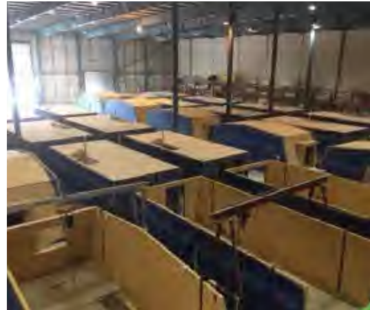
Modular construction factory, Ashford (image courtesy of Brooke Homes)
