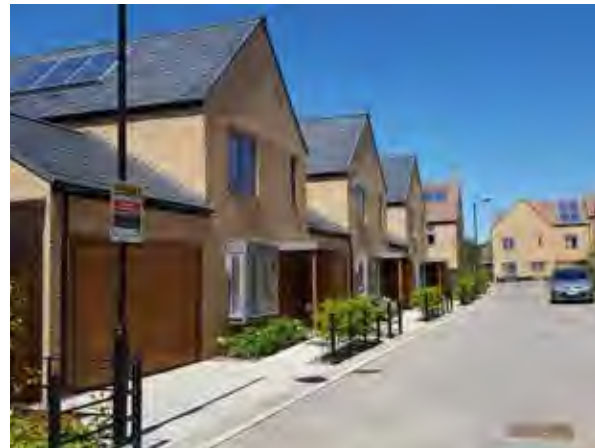
Photovoltaic panels, Trumpington Meadows, Cambridge
