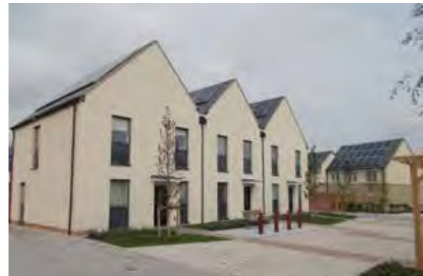
A shared surface street - NW Bicester
