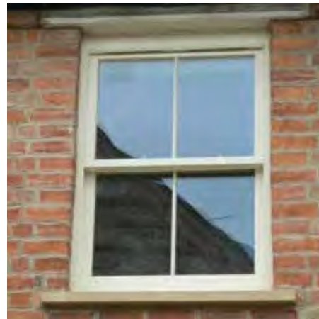
Sash window, Woodstock
