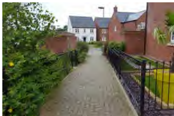
Pedestrian/ cycle cut-through, South West Bicester
