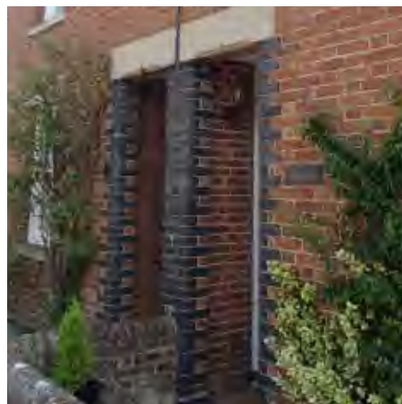
Localised brick detail around doorways
