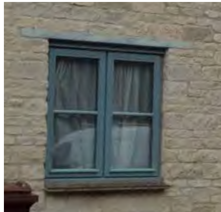
Casement window flush with wall, Bletchingdon
