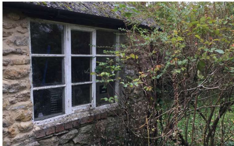
Existing ancillary building: store room window
