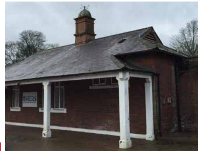
3. Concrete columns with wooden bell tower
