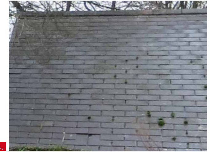
4. Low pitch slate tiles - gable ends
