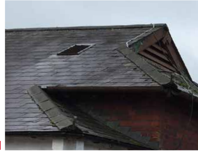
1. Low pitch slate tiles - hipped/ gablet
