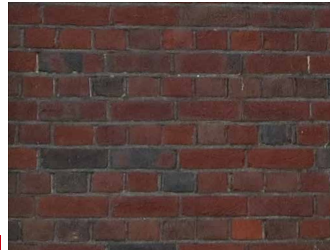
2. Dark red brickwork - English bond
