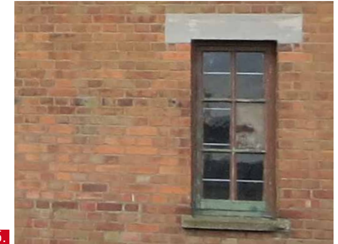
5. Light red brickwork - English bond
