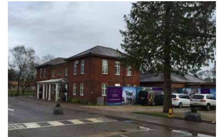
Building 52 (Heyford House)
