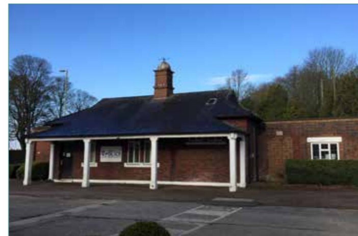
Building 100 (Guard House)
