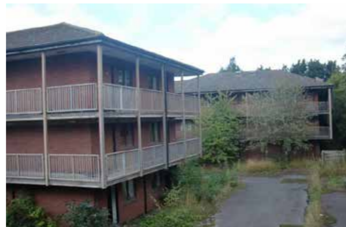
Bulding 598 (Dormitory Block)/ Hospital
