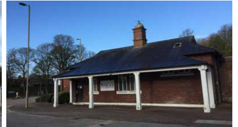
Fig.2) Building 100 - Eastern Elevation (fronting Trident Approach)
