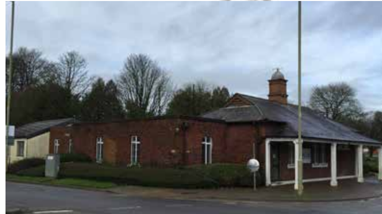
Fig.1) Building 100 - Southern Elevation (fronting Camp Road)
