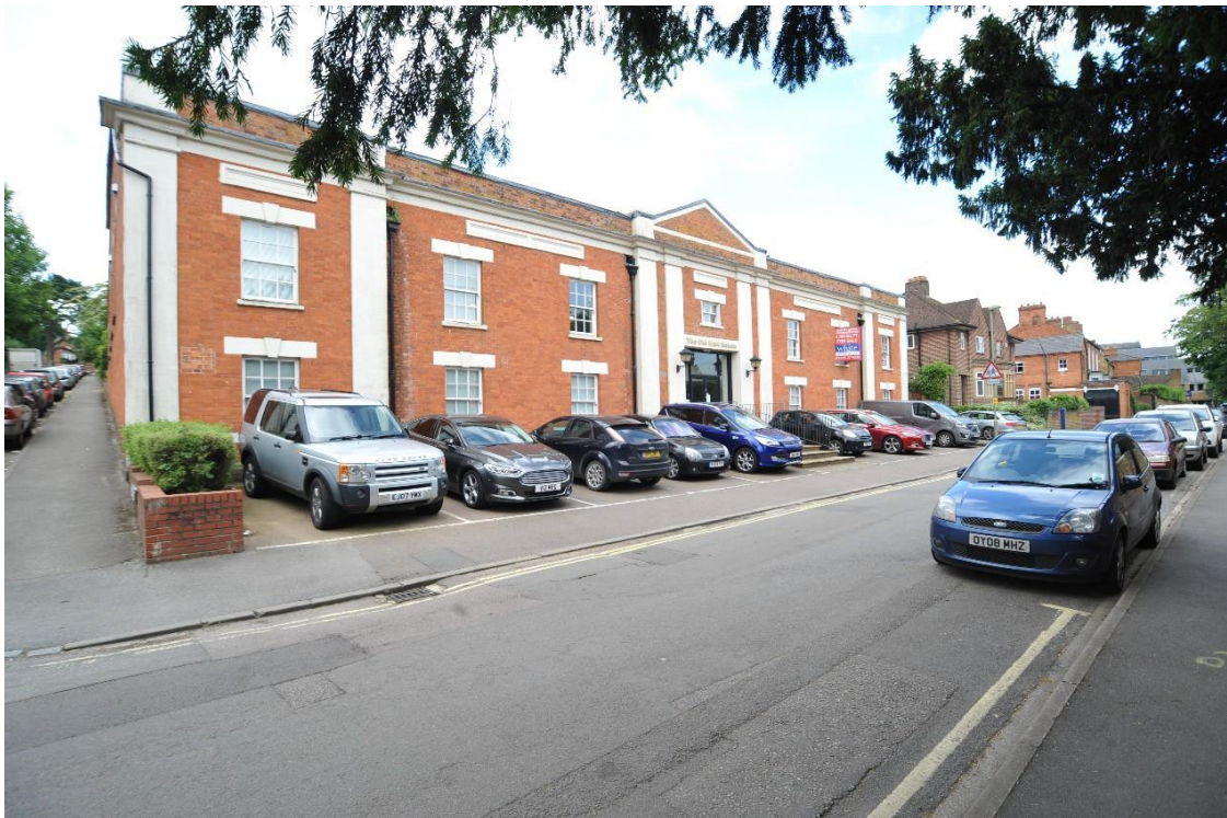
Pl.3: The front elevation from the north-east.
