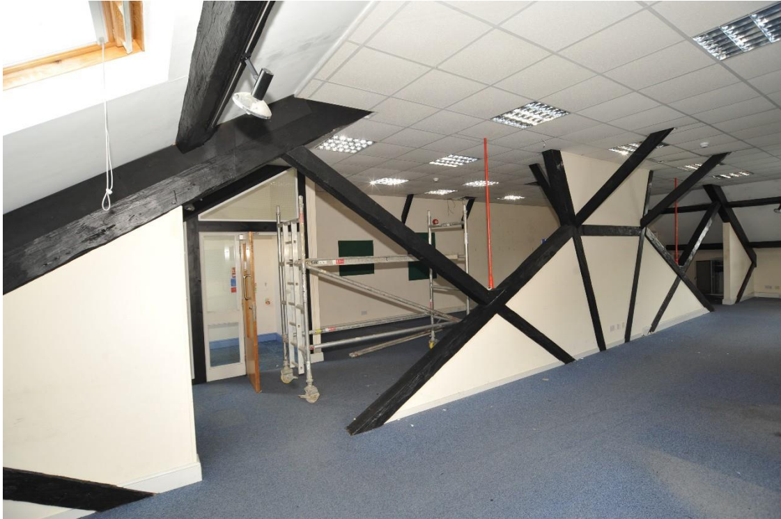
Pl.9: The exposed section of the westernmost truss, viewed from the second floor.
