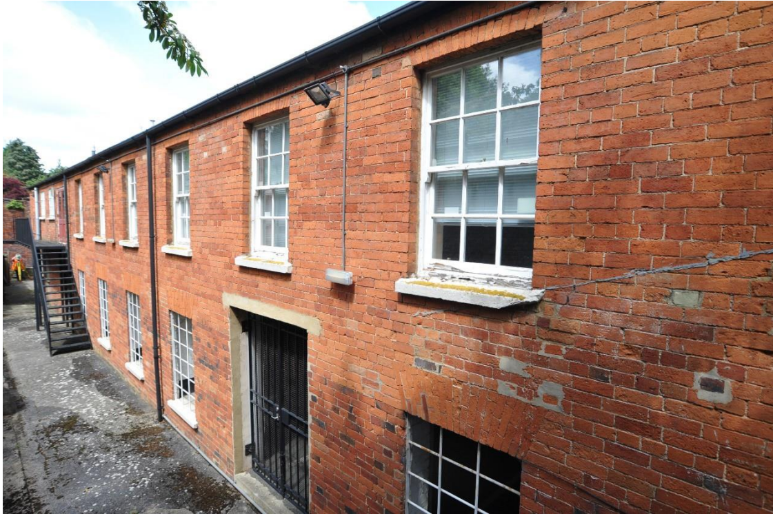
Pl.4: The rear elevation from the south-east.
