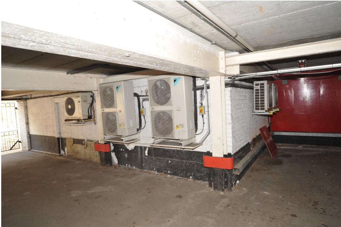
Pl.15: Another modernised portion of the ground floor.
