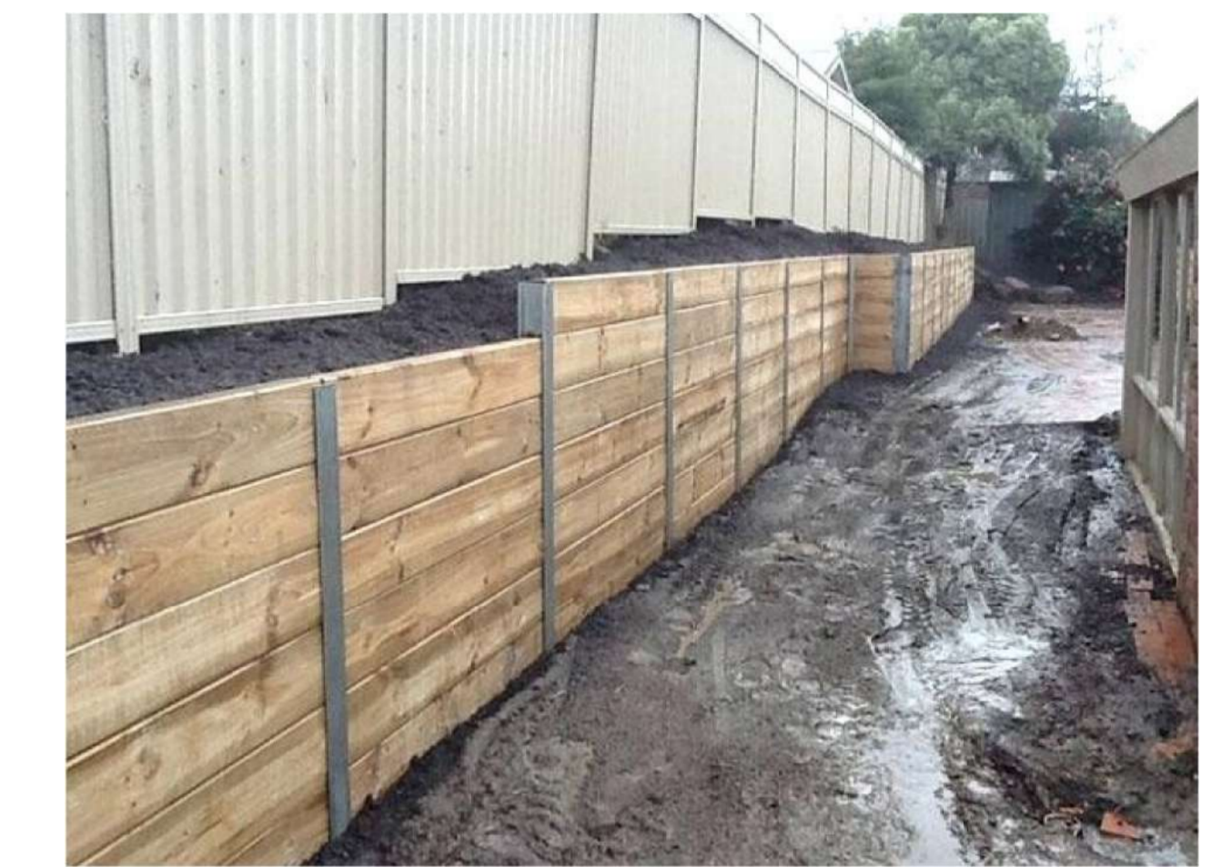
08 TIMBER RETAINING STRUCTURE 2017 around substation etc
