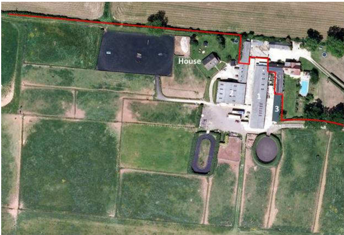
Figure 1 Aerial view of the buildings and adjacent paddocks
