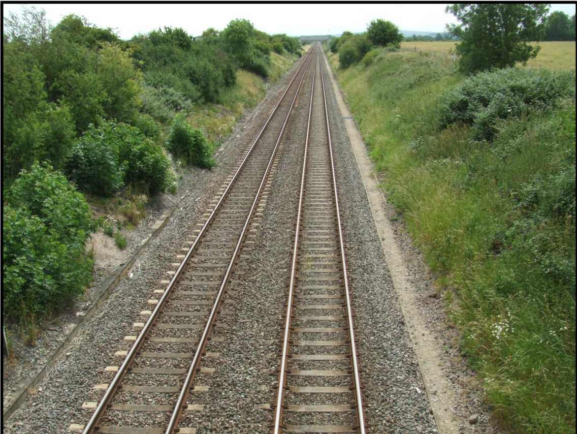
Plate 9: The London to Birmingham railway line as it passes within the cutting beneath Middleton Road to the south-west of Bucknell village
