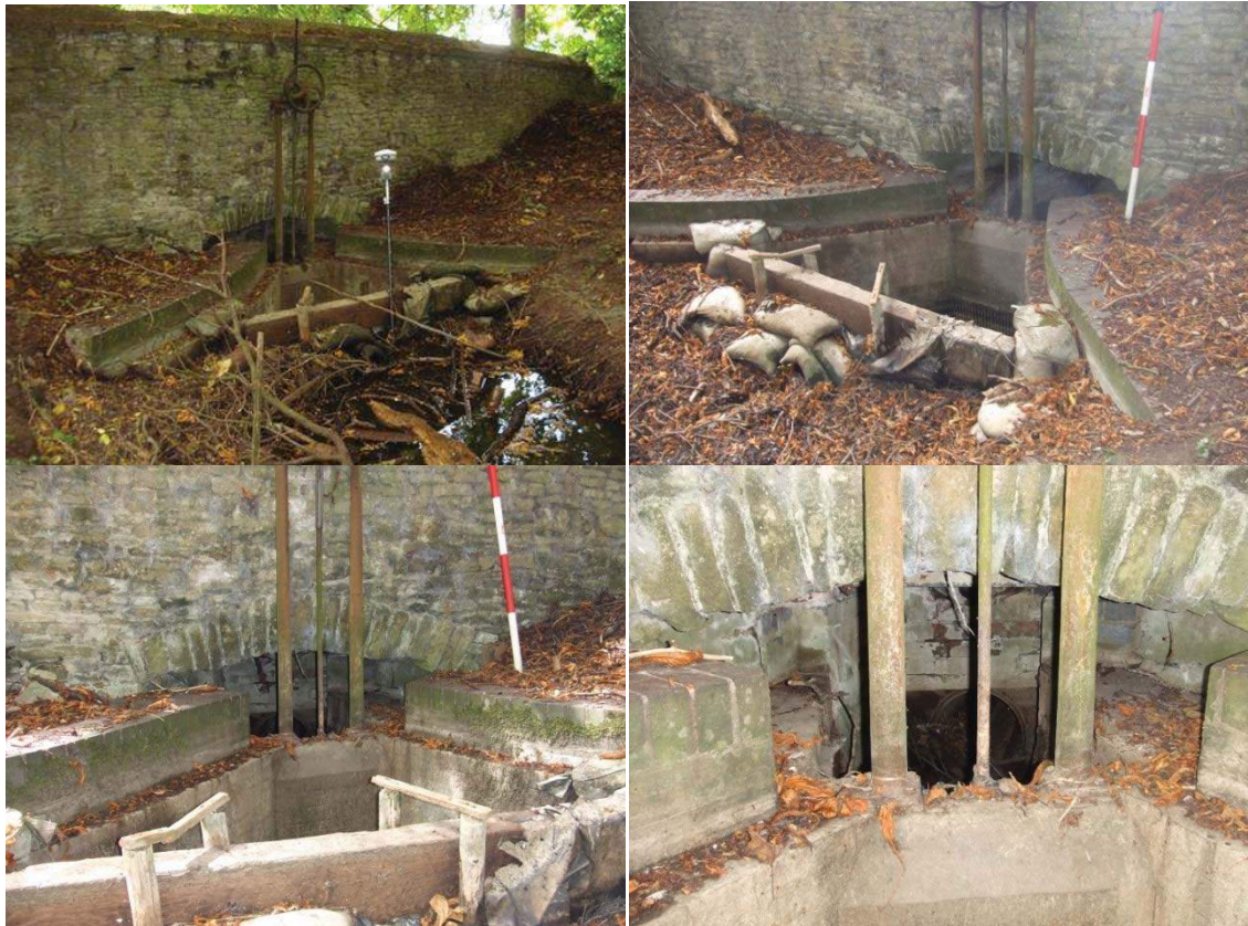
Figure 6 – Photographs of the structures at T3-356
