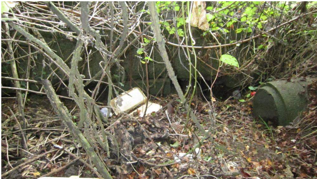
Figure 4-3 Existing Outfall under Howes Lane
