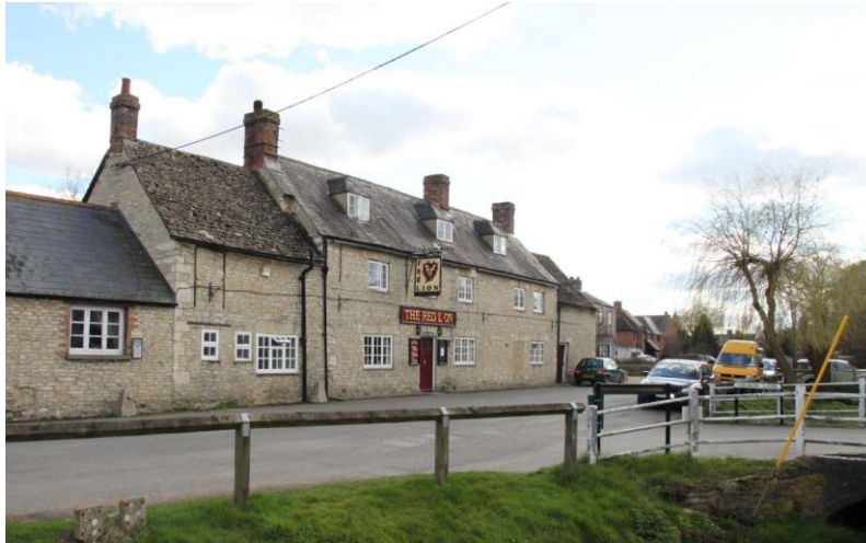
Frontage of Pub – Including bridge/ un-named watercourse opposite
