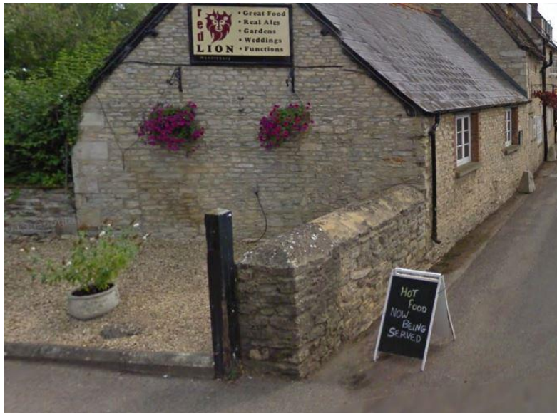
Rain Water Down Pipe discharging to road
