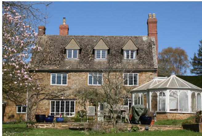
Original house with ill-suited conservatory
