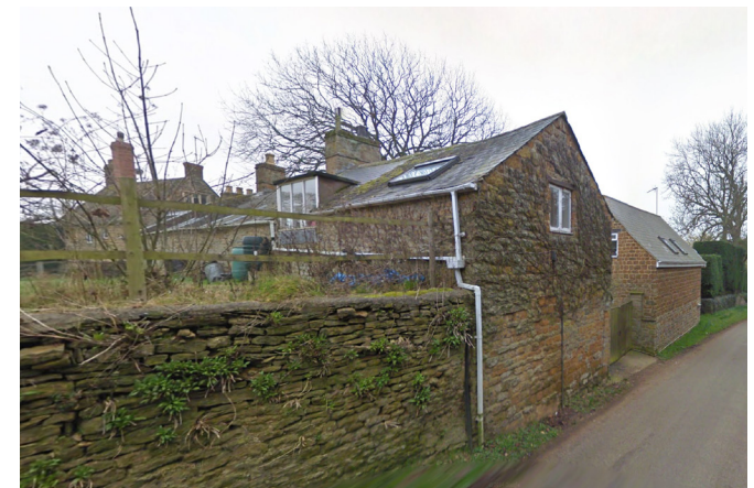
Temple Close looking south east from Temple Mill Road
