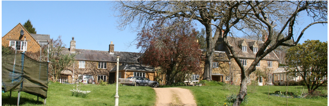
Front/South Elevation Viewed from Drive
