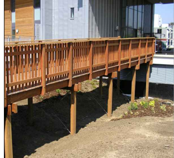
PROPOSED TIMBER BRIDGE. To be FSC hardwood, 'Woodscape Hardwood Timber Vertical Infill Bridge' or equal approved.
