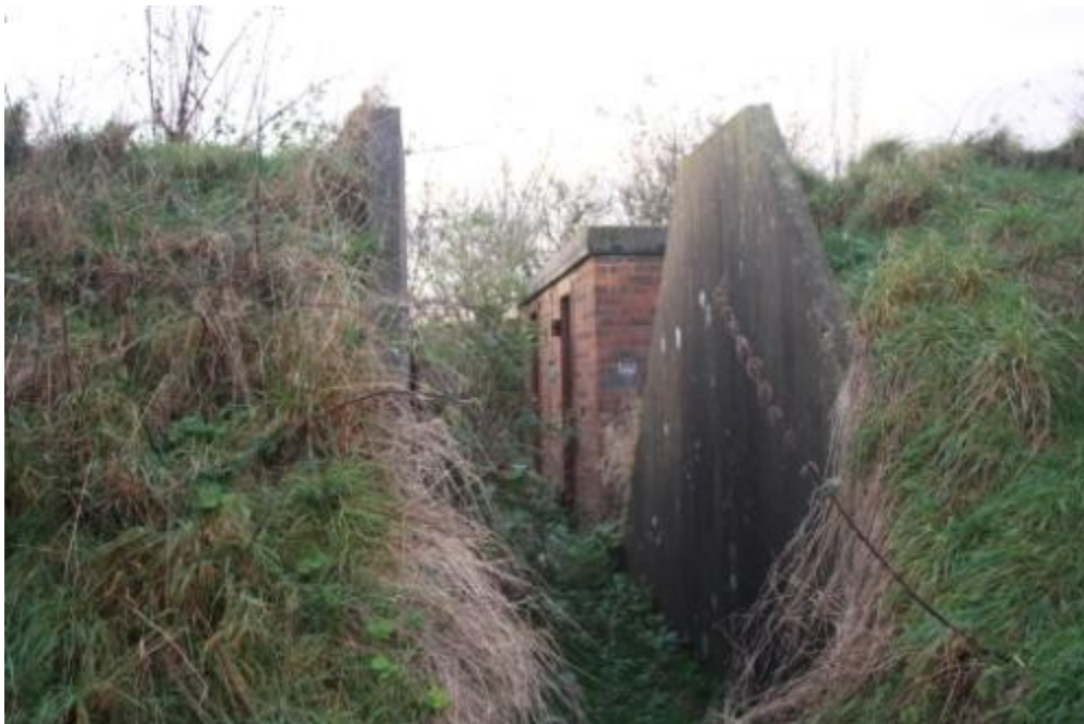
Plate 1: Typical view of one of the brick and concrete bomb store buildings protected by earth banking.
