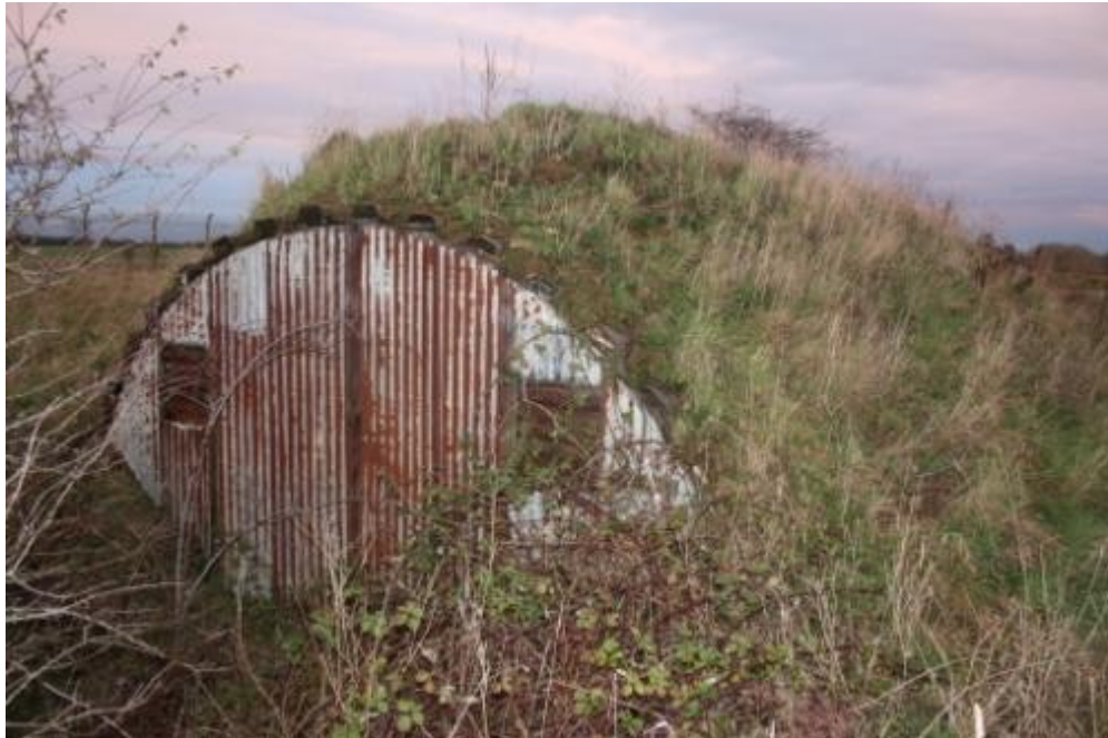
Plate 2: View of one of the curved roof corrugated steel and earth Ultra Heavy Fusing point buildings
