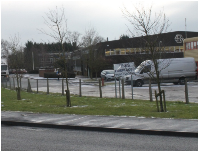
Photo 5: Employment land (distribution warehouses, Launton Road)
