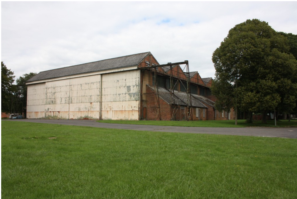
Plate 3: General view of one of the 'Type A' hangars.
