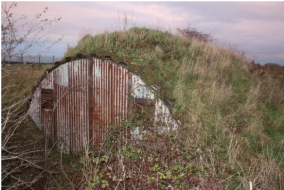
Plate 7: View of one of the curved roof corrugated steel and earth Ultra Heavy Fusing point buildings
