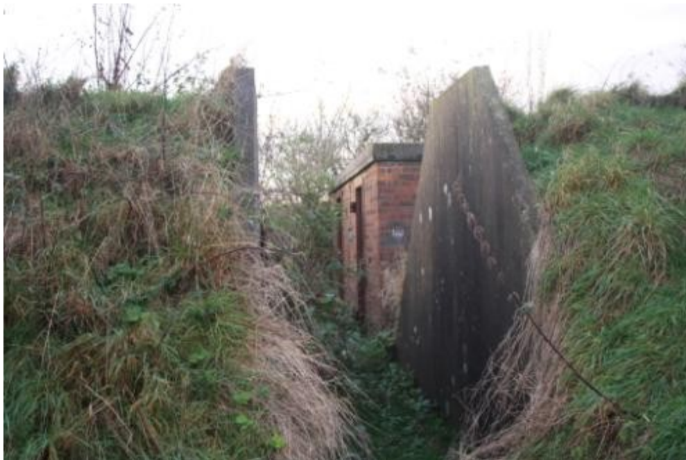
Plate 6: Typical view of one of the brick and concrete bomb store buildings protected by earth banking.
