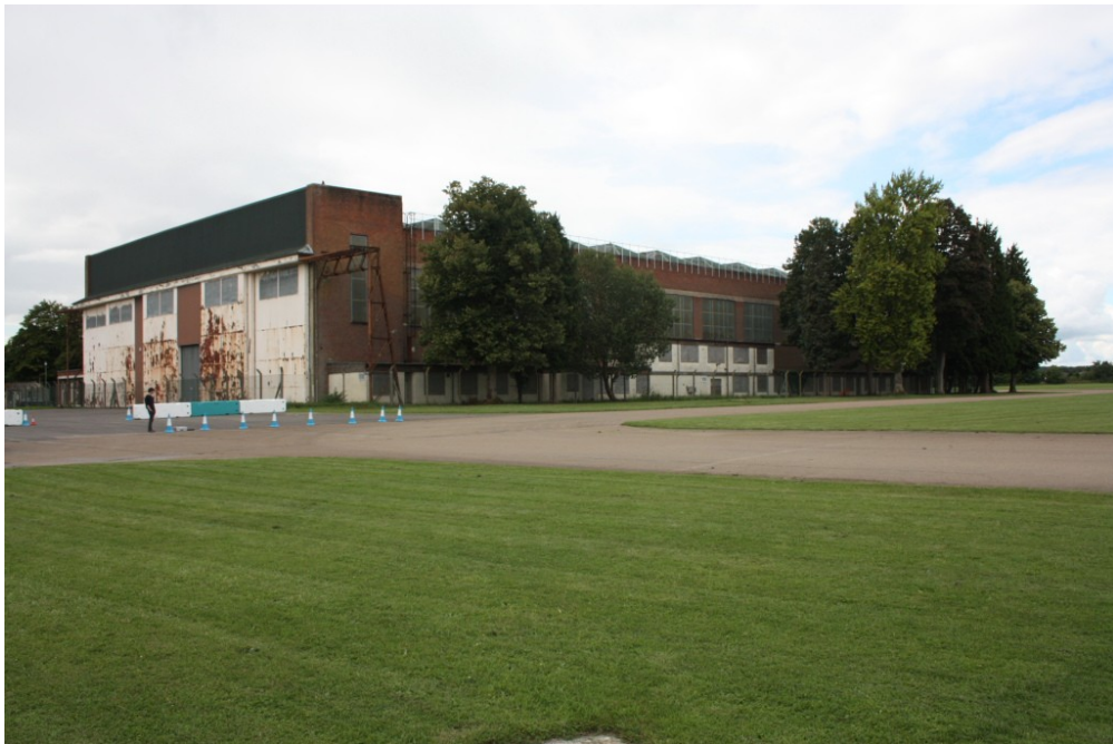
Plate 4: General view of one of the 'Type C' hangars
