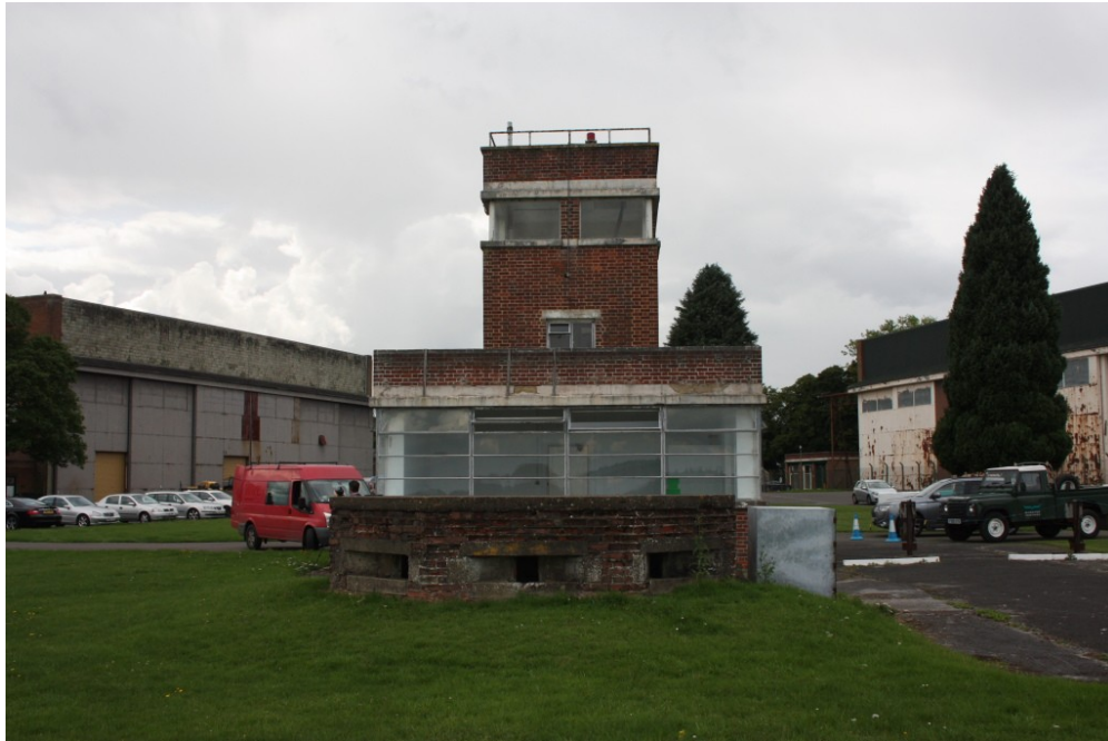
Plate 1: General view of the grade II listed Watch Tower/Office of 1934 'Fort' type design. Note brick facing and flat roof construction. Note the defensive pillbox in front and the two 'Type C' aircraft hangars to the sides
