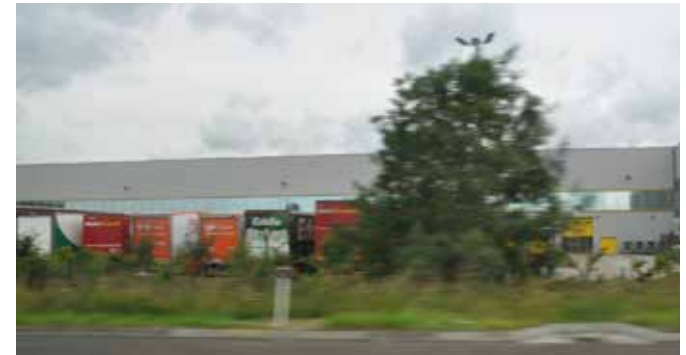
Fig 39 Amazon distribution Centre
