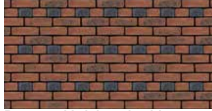
Patterned brickwork with different coloured headers
