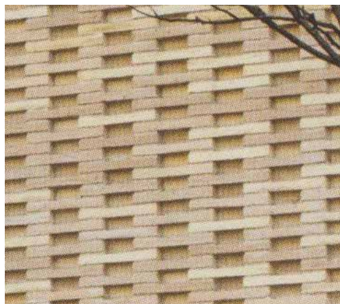
Textured brick pattern with recessed bricks
