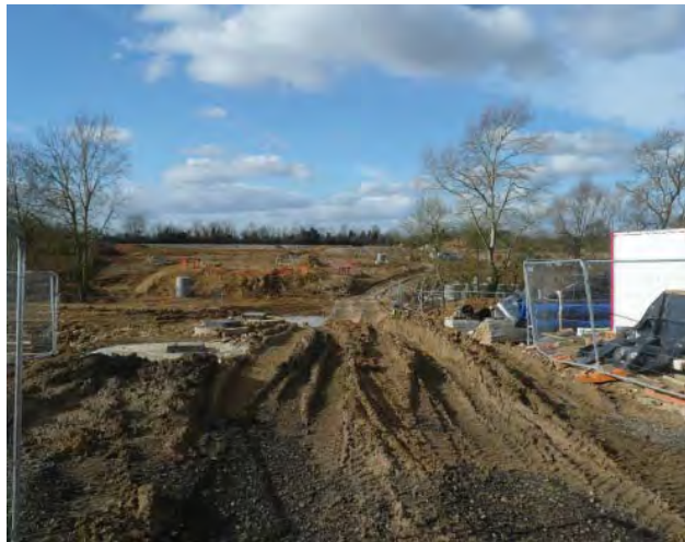
View of site looking west from street
