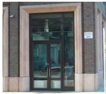
Reconstructed stone entrance surrounds
