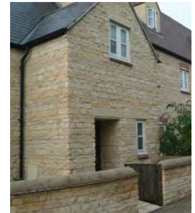
Stone houses in Bicester
