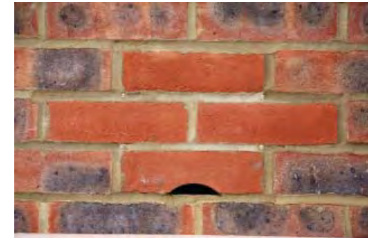
Bat box in wall
