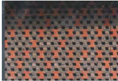
Contrast brick vent opening
