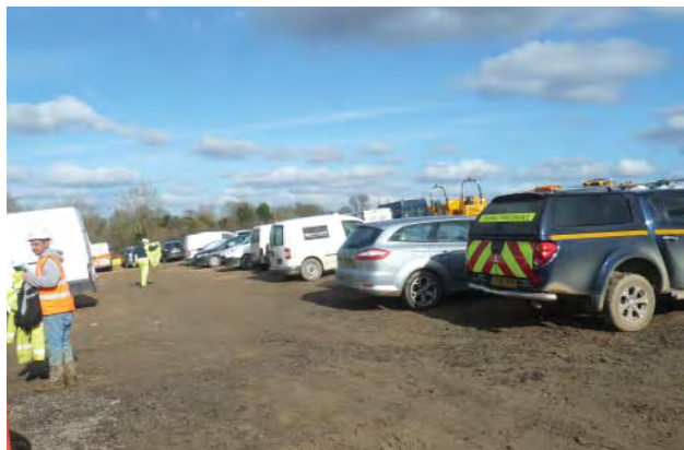
The existing site - View of the site north from the street
